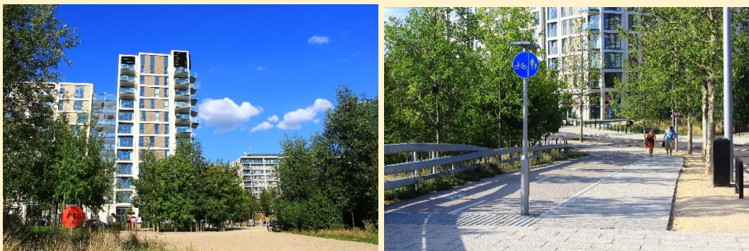
Olympic East Village, London – Taller apartments, ground floor retail and generous public open space
