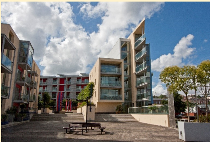
The Point, Bristol – Apartments and public space along waterfront
